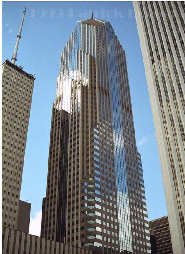
**FIGURA. 1.** Two Prudential Plaza Chicago: Hormigón 82 MPa
