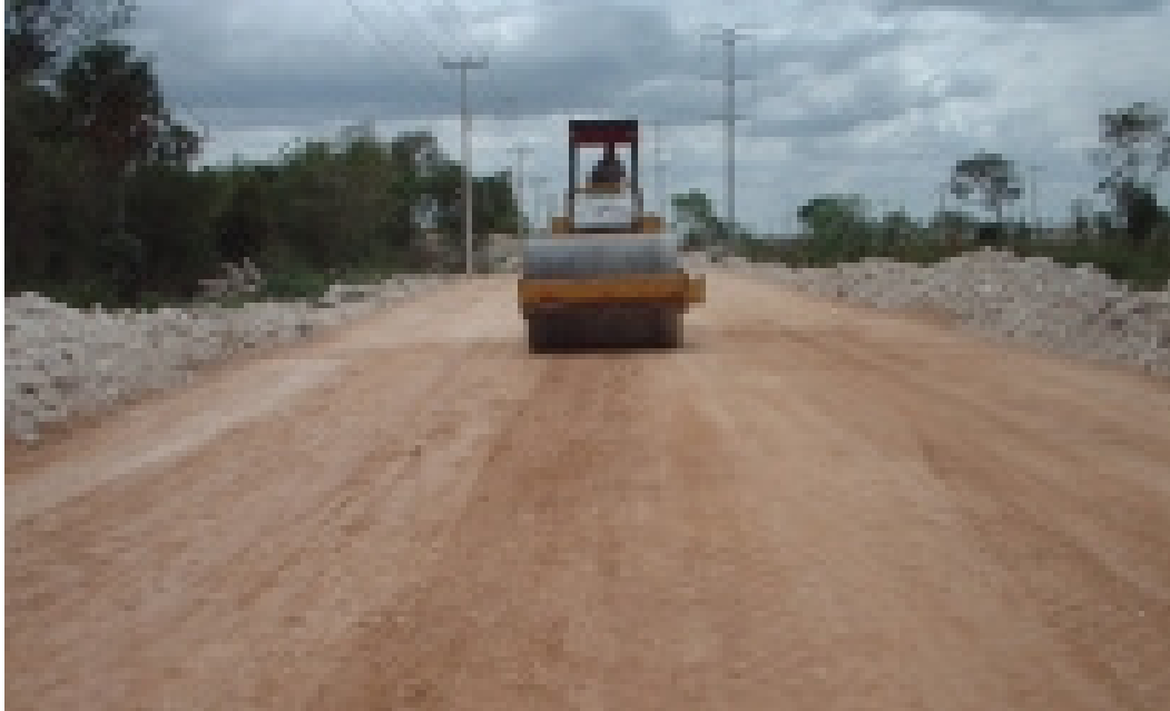
Compactado material sub-base o base
