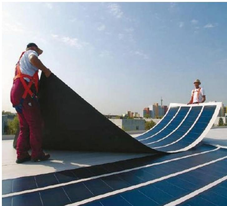
Figura 3.20. Paneles Flexibles
