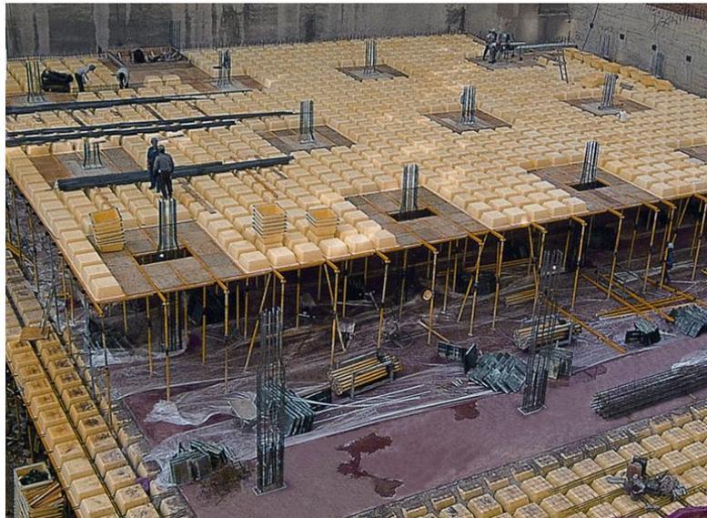
Fig 3.5 Encofrado recuperable
