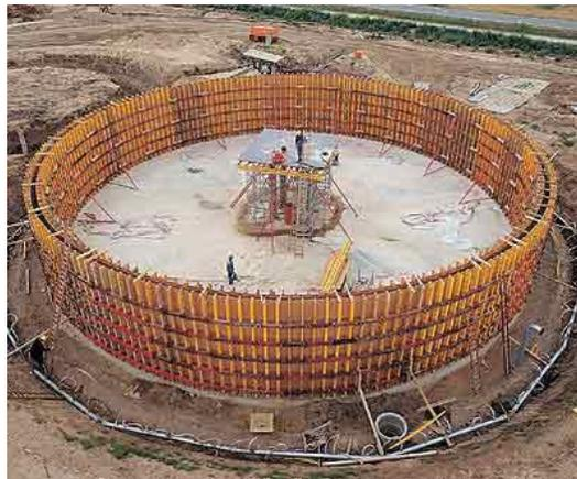
Fig. 4.30 Muros curvos
