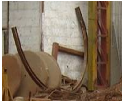
FIGURA 4.17 E4,5,6,7: VIGA CURVA
