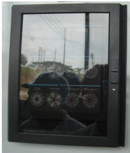
Figura 1.8. General Electric 735 Feeder Protection
