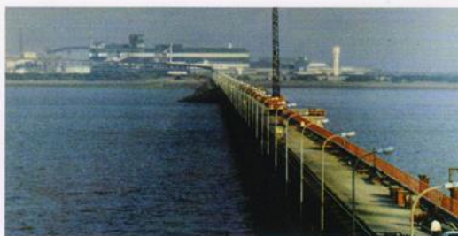
Fig. 4: Straight portion of pipe conveyor at jetty
