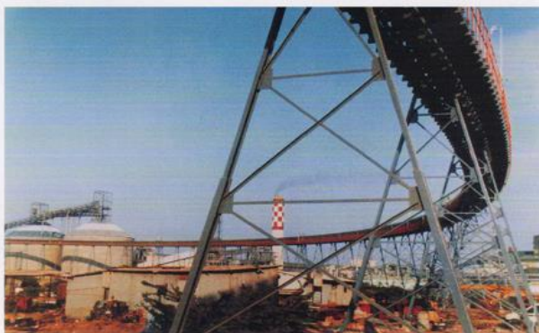
Fig.1: 3.2 km long pipe conveyor at Birla Copper
