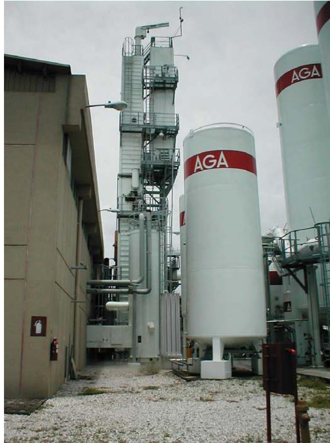
**FIGURA 2.8. LA DOBLE COLUMNA LINDE DE PLANTA ASU**
