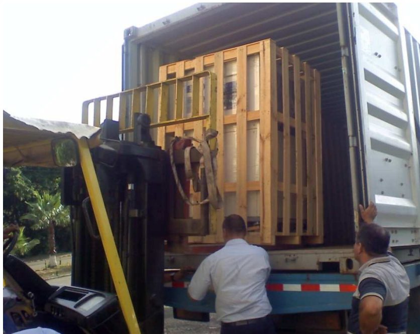
FIGURA 3.8 INGRESO DE CHILLER CHUTING.
