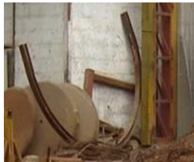
FIGURA 4.17 E4,5,6,7: VIGA CURVA
