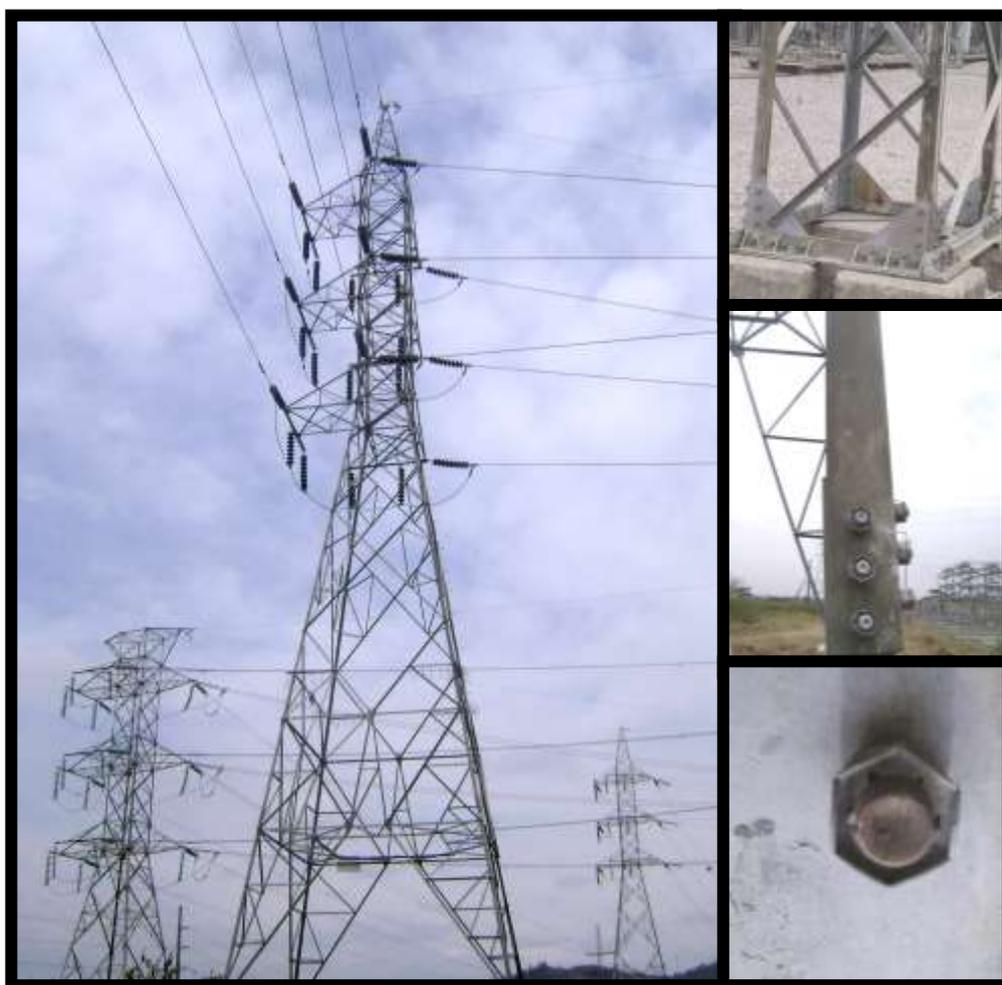
**FIGURA 1.2 PARTES AFECTADAS POR LA CORROSION**
