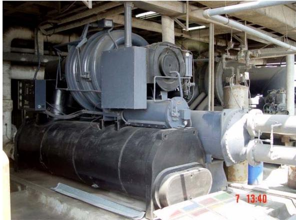
**Figura 1.3.** CHILLER CENTRAVAC MARCA TRANE
