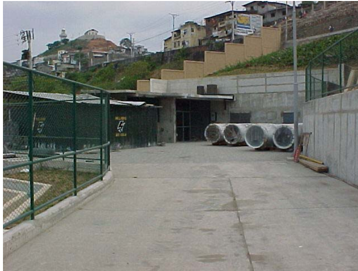
Figura 4. 13 Central de Control
