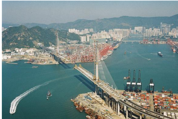
Figura 2.13: Puente Stonecutters-Hong Kong
