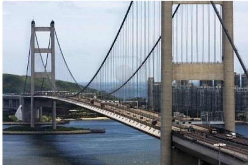
Figura 2.12: Puente Tsing Ma-Hong Kong
