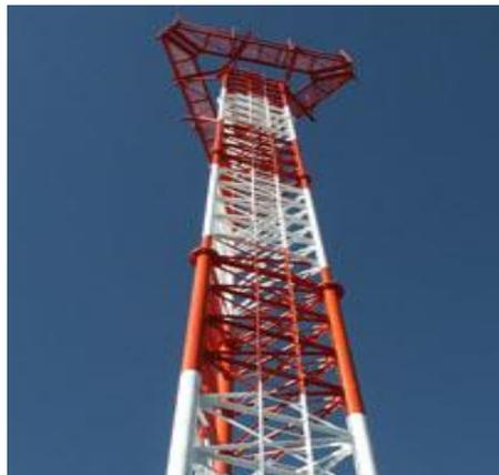
Figura 2.6 Torre autoportada triangular
