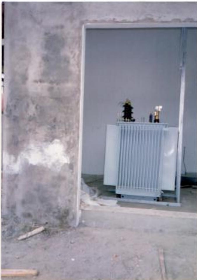
FIGURA 5.3 TRANSFORMADOR PRINCIPAL
