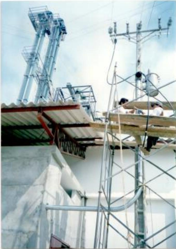
FIGURA 5.1 ESTRUCTURA DE ACOMETIDA AISLADA
