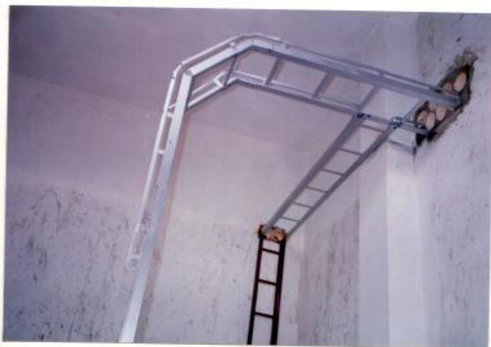
FIGURA 5.11 CRUCE EN PAREDES DE ELECTROCANALES
