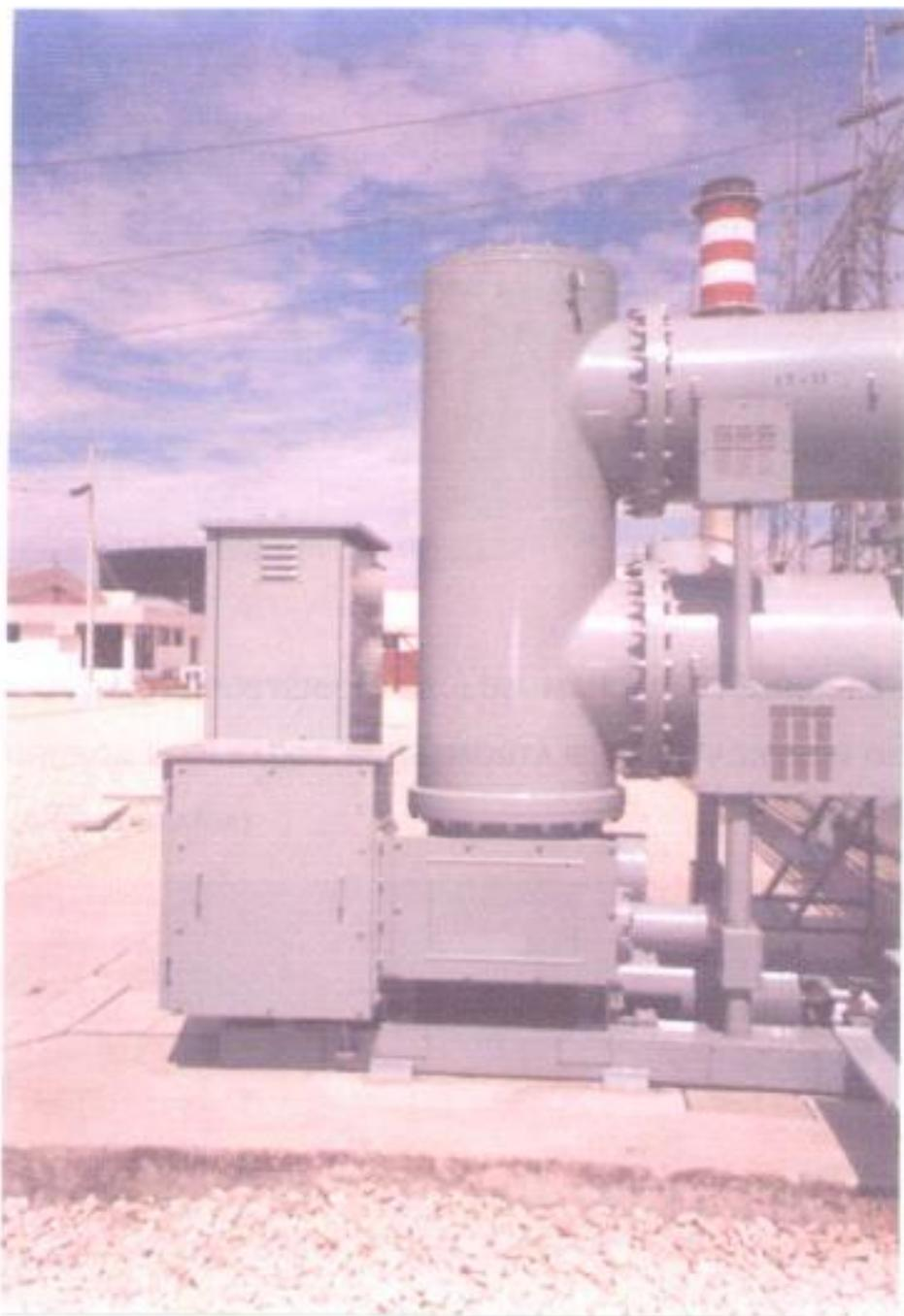
**FIG. 20 VISTA LATERAL DISYUNTOR POSICION PVG 2 138 KV S/E
