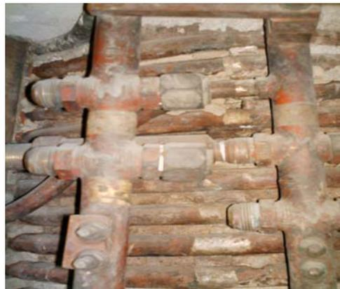
**FIGURA 1.15. CONECTORES (1" N.T.P.) DE CUBA B**
