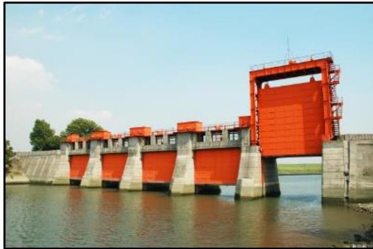
Figura 1.7: Compuerta deslizante vertical. (Iwabuchi Sluice Gate, 2020)
