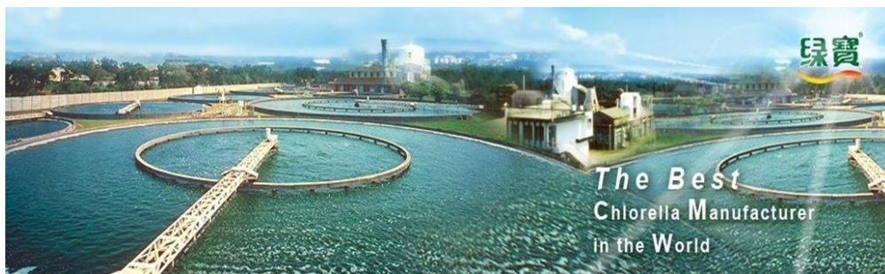
Figura 1. 11 Tanques circulares. [Manufacturing, 1964]
