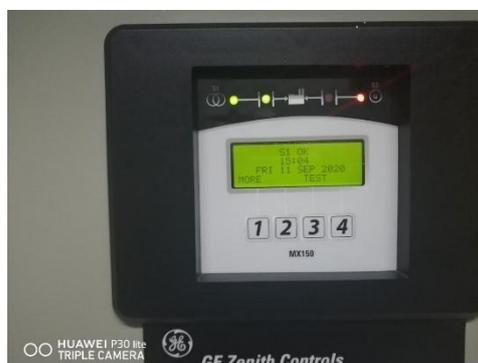
Figura 1.2 Panel de Control MX150 – Vista Frontal
