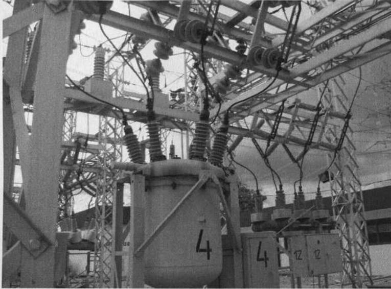
Fig. 11. Oil Circuit Breaker u OCB.
