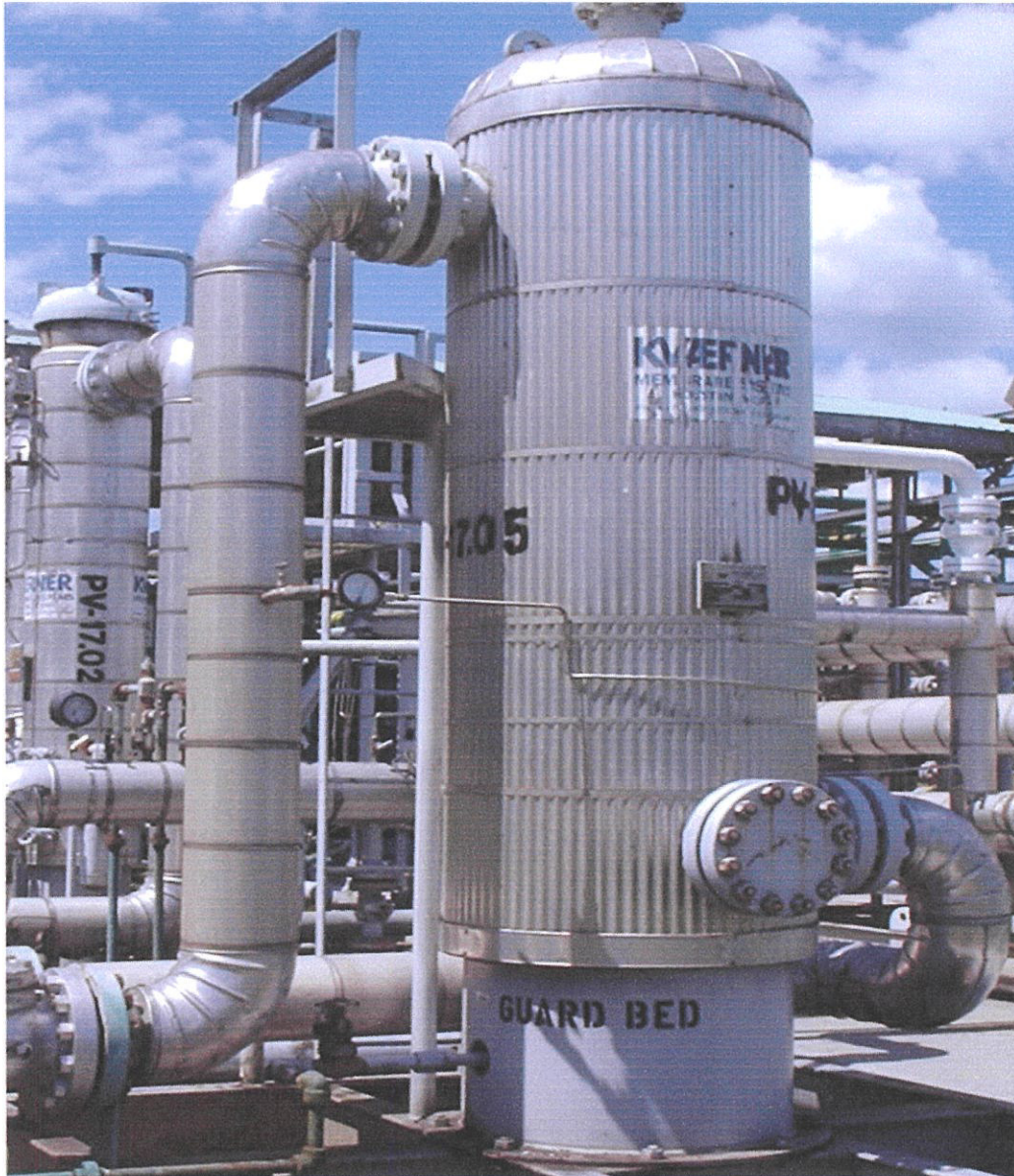
FIGURA 2.9. GUARD BED (PV-17.05)
