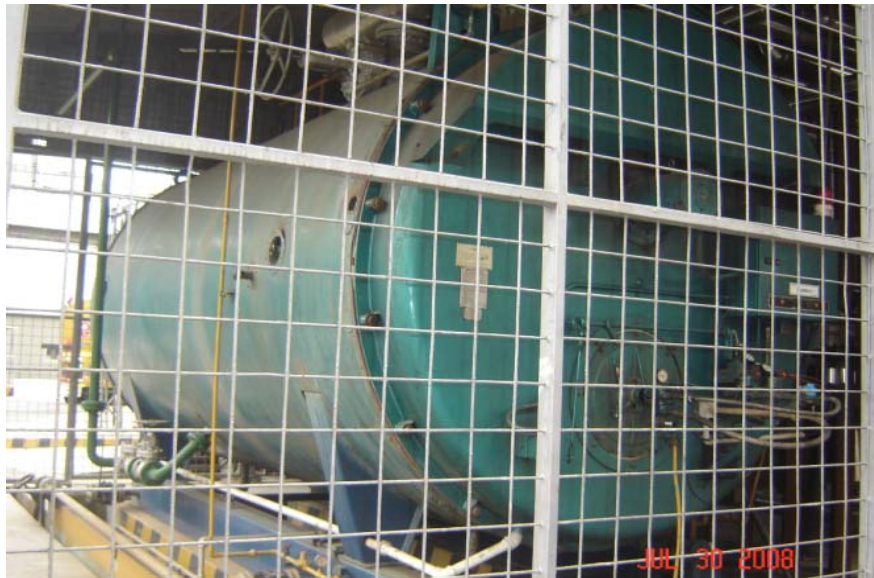
FIGURA 2.1 CALDERO CLEAVER BROOKS
