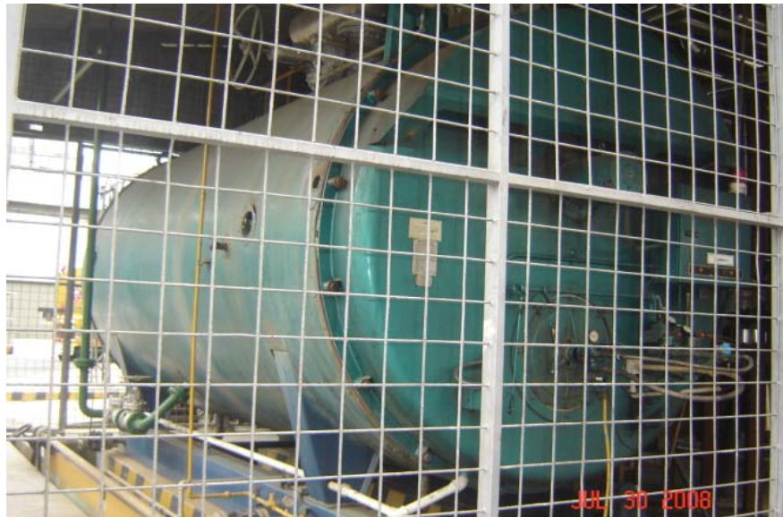
FIGURA 2.1 CALDERO CLEAVER BROOKS
