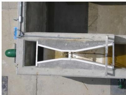
TRANSMISOR SENSOR DE CAUDAL EN CANAL PARSHALL DE SALIDA
