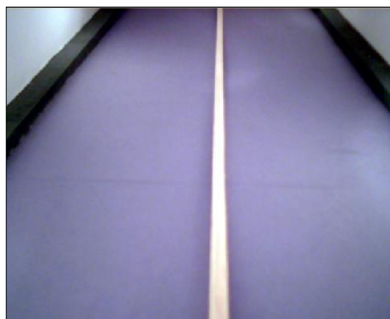
Panel central – interior túnel
