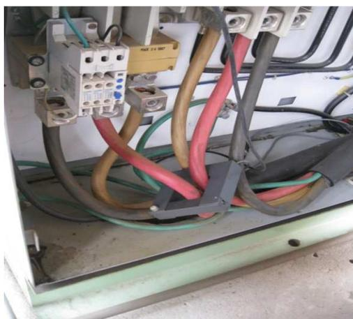
**FIG. 3.6 TRANSDUCTOR DE CORRIENTE**
