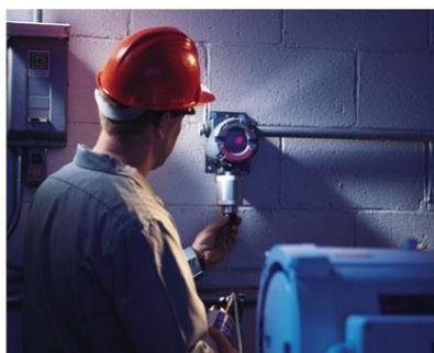
**FIGURA 2.9 MONITOR FIJO INSTALADO**
