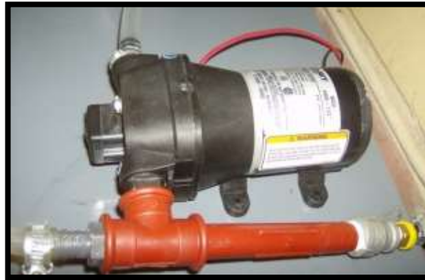
Figura 4.3 – Bomba y bypass
