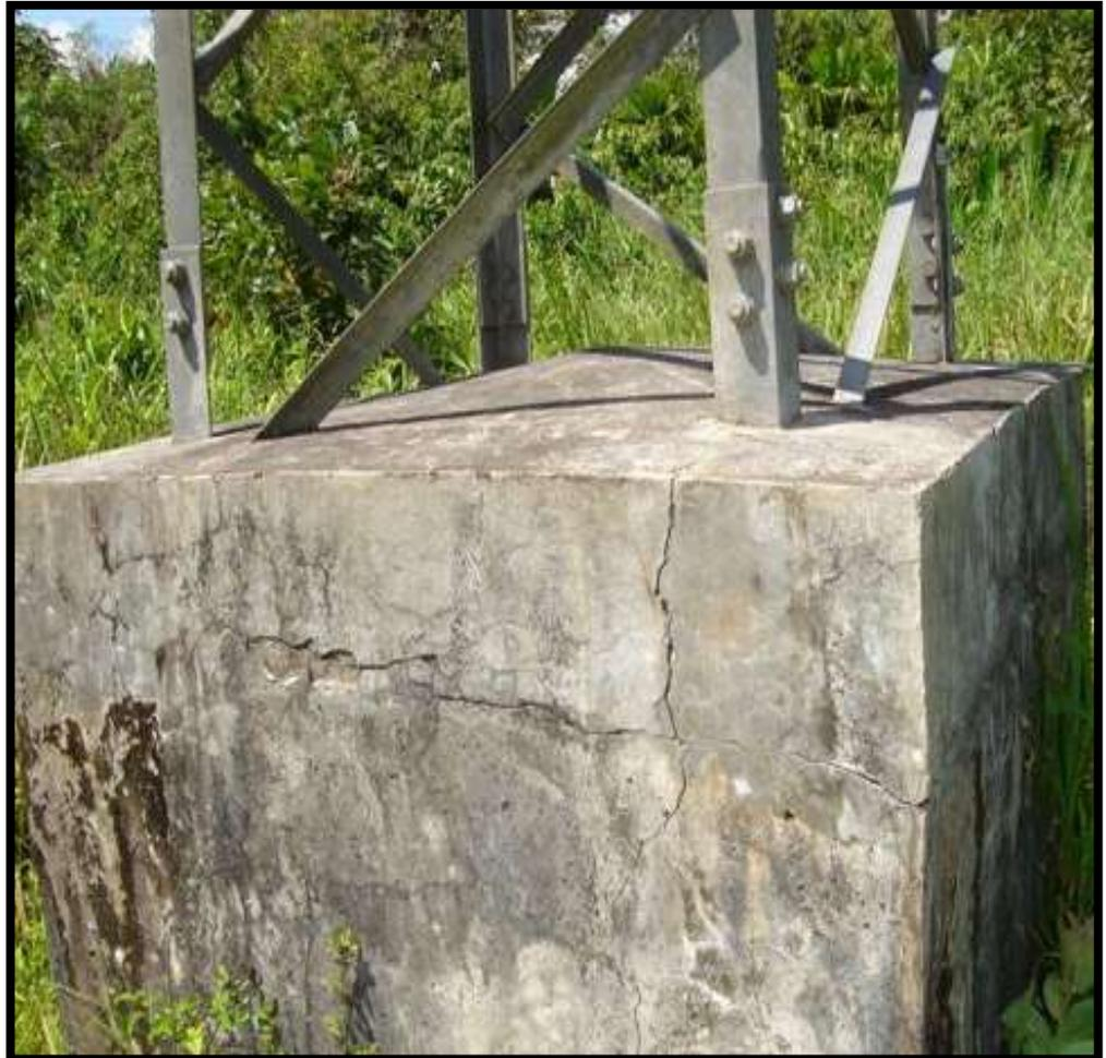
**FIGURA 1.3 CORROSION DEBIDO A FISURAS EN BASE DE
