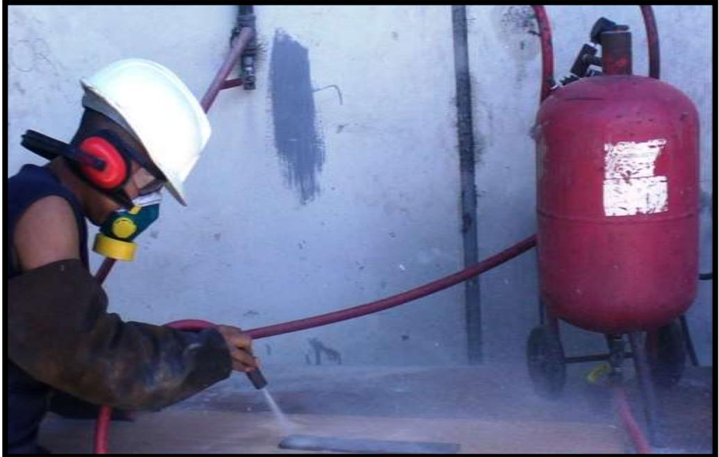
**FIGURA 2.5 LIMPIEZA CON SANDBLASTING (ARENA A PRESION)**
