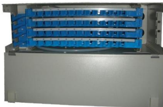
Figura 3.3 ODF Huawei [20]
