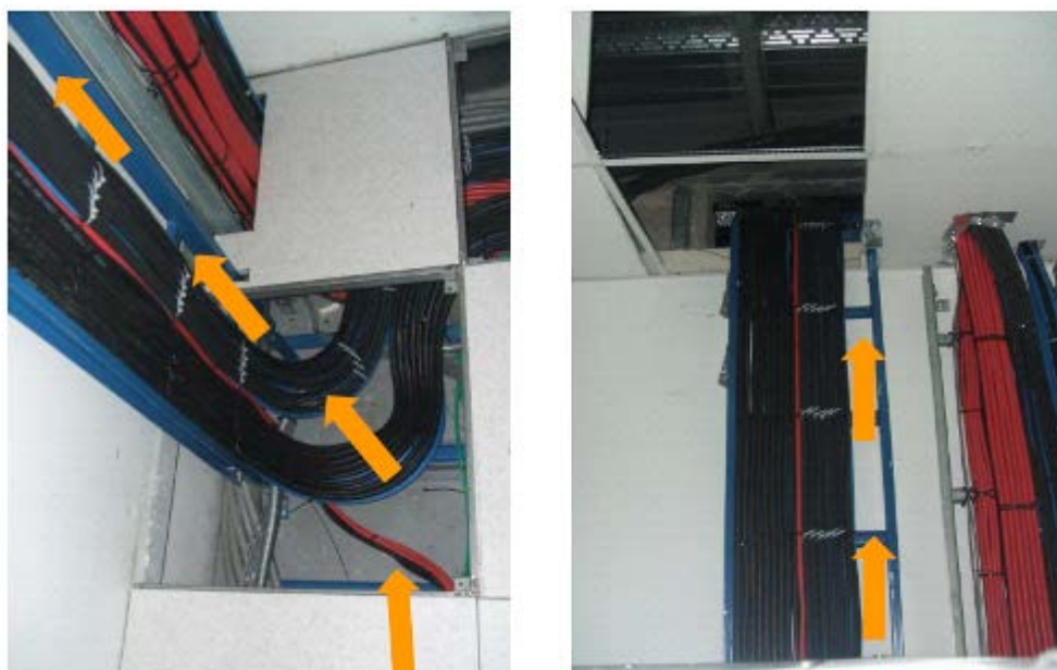
FIGURA 4-13 CABLE DE ENERGIA RECORRIDO VERTICAL
