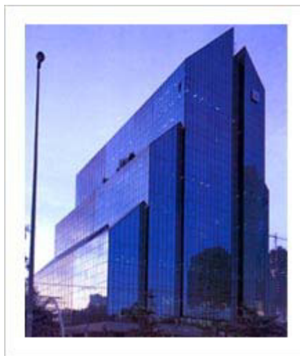
Figura No. 2-1: International Water Services-Rumania
