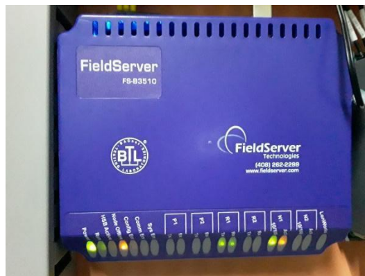
Figura 1.16 Convertidor / Gateway Bacnet IP – Modbus RTU
