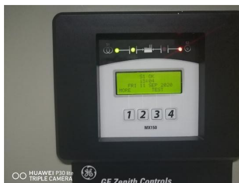
Figura 1.2 Panel de Control MX150 – Vista Frontal
