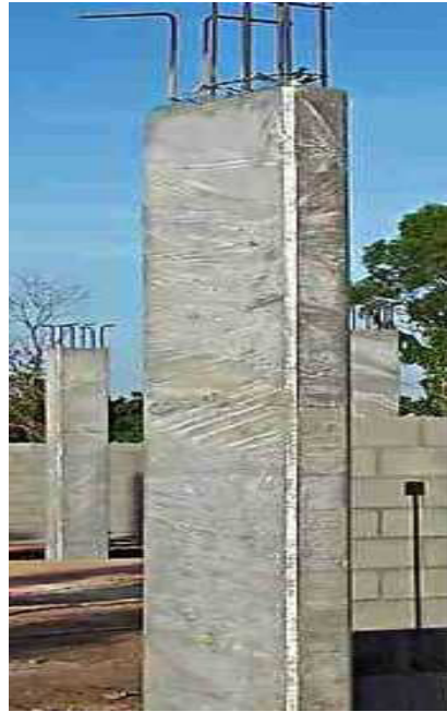
FIGURA 3.6 CURADO DE COLUMNAS USANDO PLÁSTICO http://www.builderbill-diy-help.com my website
